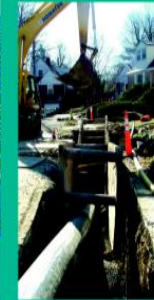
Neighborhood Construction Projects
